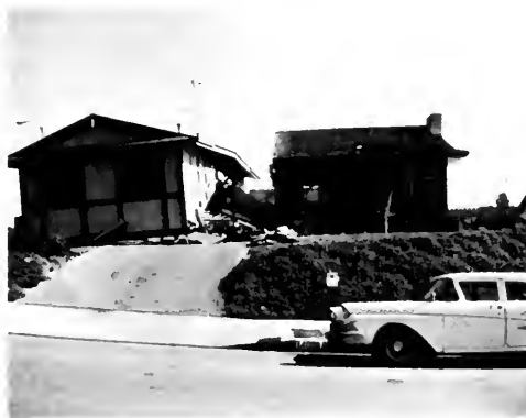
Photo 9. Left section of this dwelling was originally two stories (over garage) and attached to one-story section on right. Garage areas normally have comparatively little bracing.
